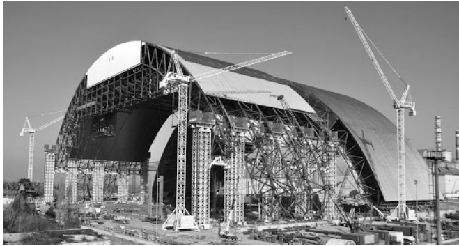
Fig. 28. Installation of confinement structures
