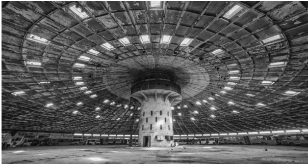
Fig. 27. Roof of bus fleet
